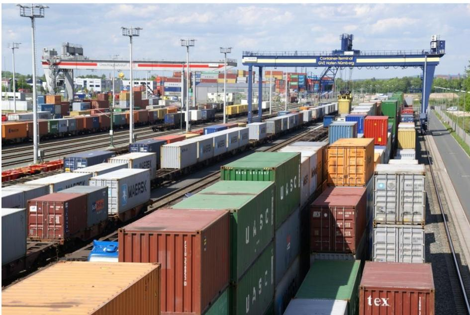
THE container terminal for the Nuremberg region in the heart of bayernhafen Nürnberg: Goods are transferred using intermodal transport between rail, water and road by ten loading sidings, four rail gantry cranes and a total capacity of 533,000 TEU per year.
